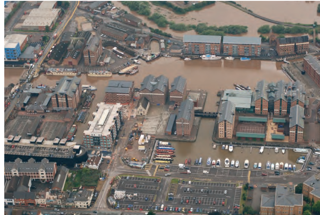
Flooding in Gloucester Docks, 2007
